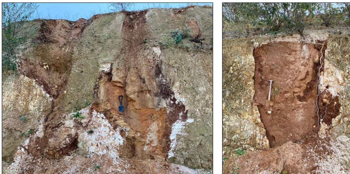
Figure 36. Dissolution pipes infilled with orange-brown sand and lined with darker brown flinty clay, Newport Chalk quarry. Hammer and spade c. 0.35 m high.
