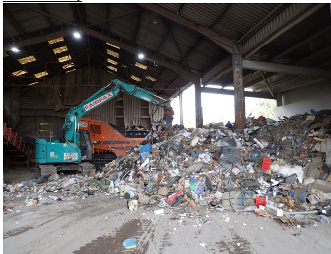
Image 6 shows combustible non-hazardous waste spilling out of the bay
