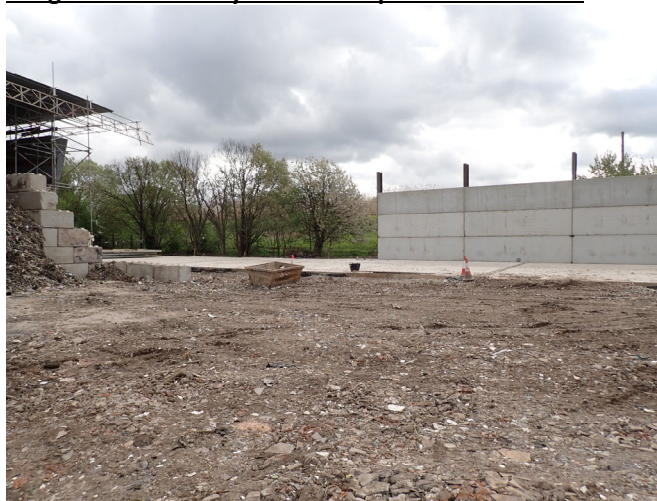
Image 2 shows newly installed impermeable surface
