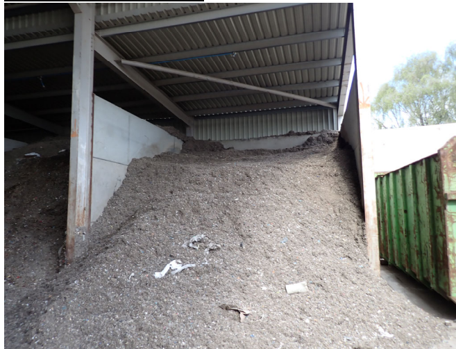
Image 4 shows combustible waste without 1m free board and spilling out of the bay
