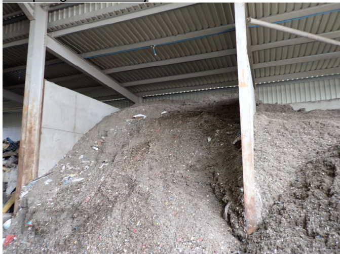
Image 5 shows combustible waste without 1m free board and spilling out of the bay
