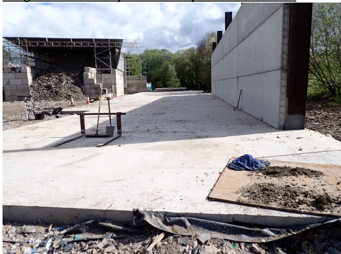
Image 1 shows newly installed impermeable surface
