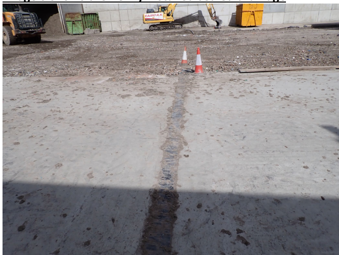
Image 3 shows the newly installed sealed drainage
