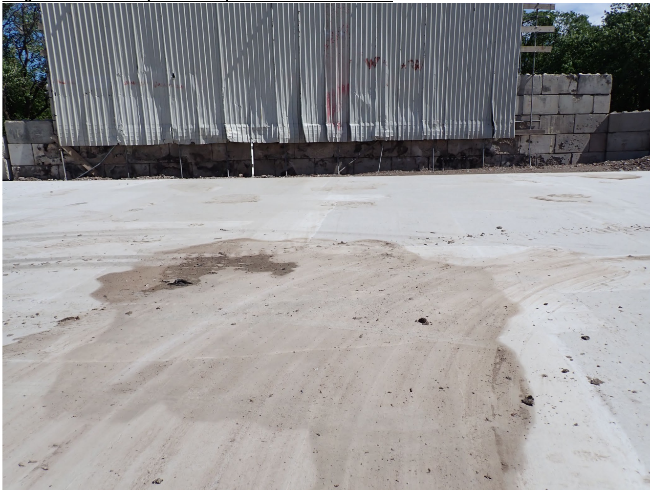
Image 1 shows the newly installed impermeable surface in Area 3
