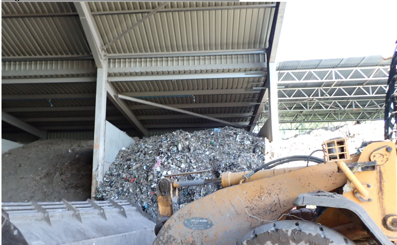
Image 2 shows shredded waste and fines without a 1m freeboard
